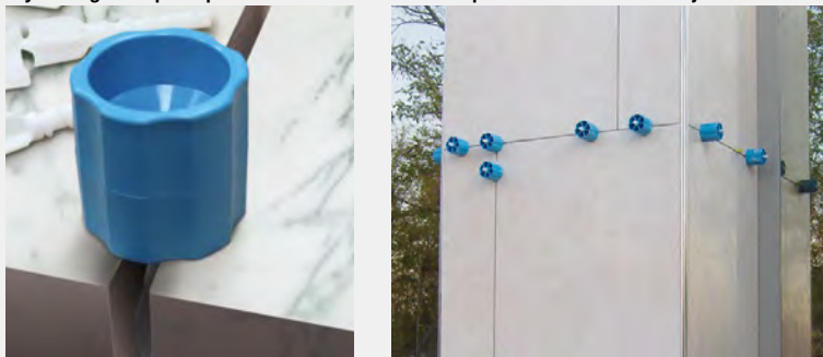
By turning the cap it is possible to level a thickness of up to 40 mm with an 8 mm joint.
