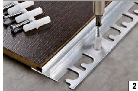
2) Fix and/or glue the base to the floor.
