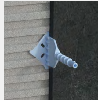
Linear leveler installation.
