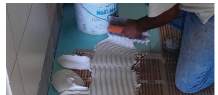
Incorporating AHT grid into a MARMOFLEX or NOVACOL FINE FLEX adhesive layer depending on the application
