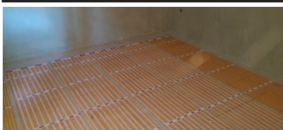
Installation of AHT electrical grid on substrate primed with PLANO CONTACT
