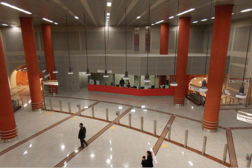
ATHENS & THESSALONIKI METRO STATIONS BONDING & GROUTING OF NATURAL GRANITE & CERAMIC TILES MARMOFLEX, NOVACOL FLEX, NOVAGROUT, PU 500, NOVACOLOR HNR
