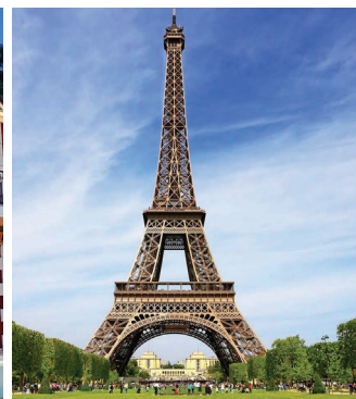
Offices in the Eiffel Tower
